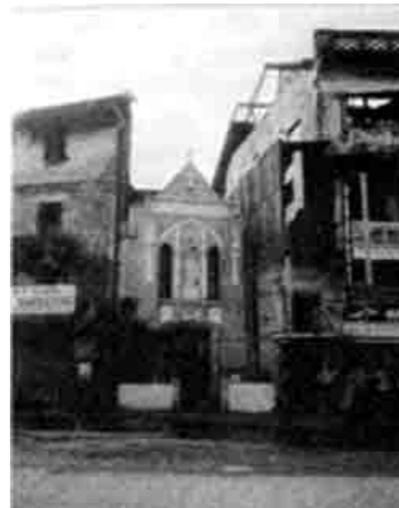
January to December 1835 - Hill Street Academy at St. Pauls Church Wolvehdal - back verandah.
